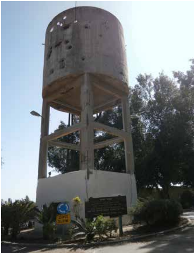
Fig. 5 Water tower in a kibbutz
